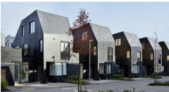
Innovative housing types at Newhall, Harlow
